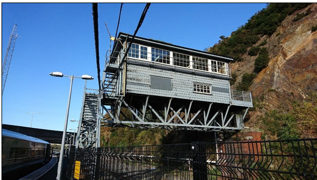
Plate 15.6 Signal box (RPS 571), facing west
