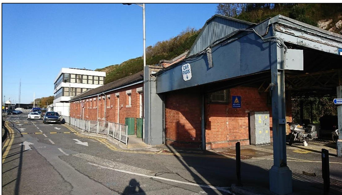
Plate 15.4 Railway Station (NIAH 22500032), facing northwest
