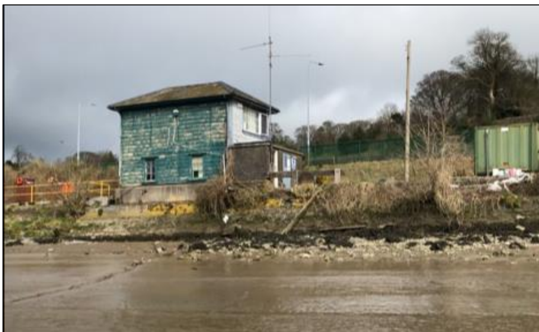
Plate 15.11 Signal box to the northwest of the proposed development
